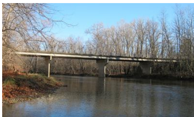
Greenhill Road - 2 lane
