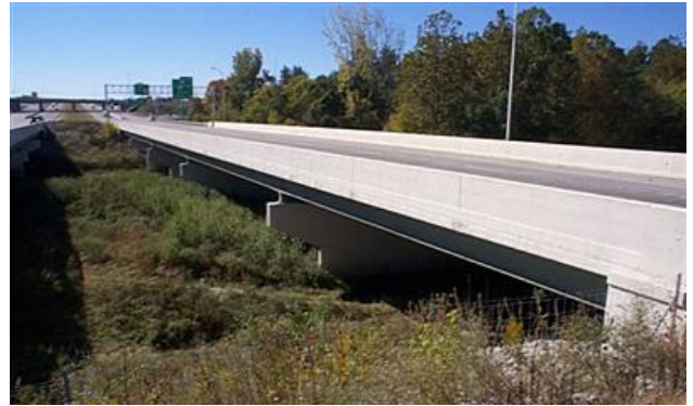
I-69 - Dual 2 lane bridges
